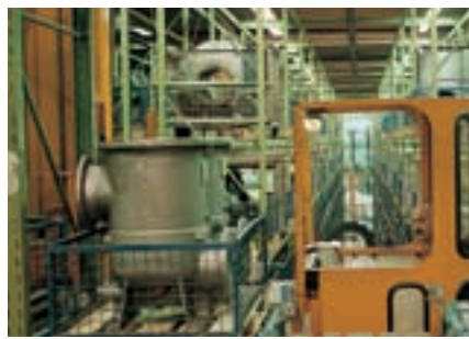
Modern storage and logistics systems support smooth and effective production.
