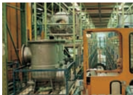
Various storage and logistics systems support smooth and effective production.
